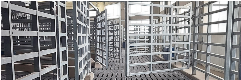
“This new barn design was based on industry-leading technology and humane methods. With no sharp corners, there’s a distinct flow through the barn, in a herringbone pattern, which doesn’t require animals to make 90-degree turns,” explains Duane Eichenlaub.
