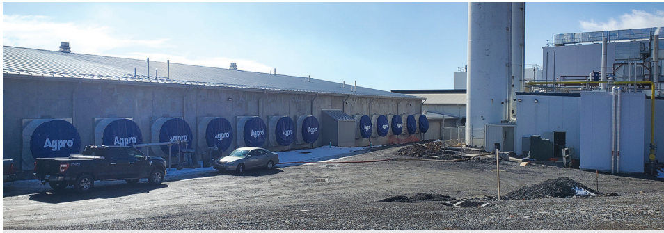
The new barn measures roughly 40,000 sq. ft. Animal welfare is paramount in the design of the barn. There are 15 fans – each nine feet in diameter – as part of the design to ensure proper air circulation and ventilation in all weather conditions.
