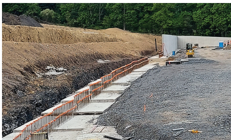
This is the eastern view of the tier II retaining wall currently under construction. This retaining wall is one of three that will enable level ground for placement of buildings and tanks.
