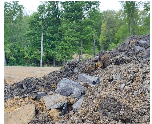
This pyritic shale must be hauled off-site and replaced with suitable material — a necessary activity that has contributed to increased truck traffic as well as added to our project schedule.
