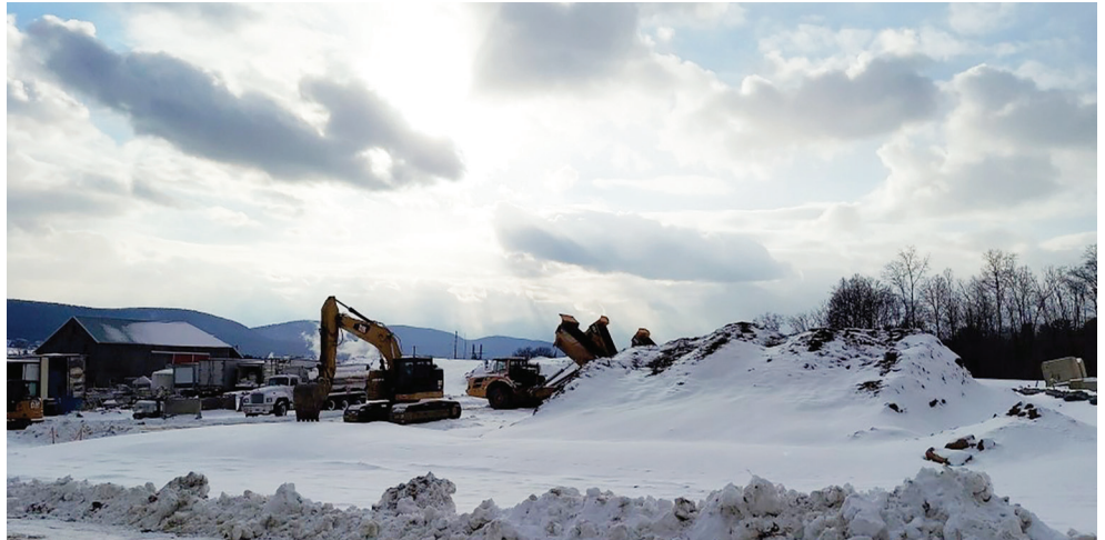
The heavy equipment sits idle amidst the snow and frigid temperatures at the Nicholas Meat Sustainable Resource Facility site. However, there’s plenty of activity happening behind the scenes as materials and supplies are secured and plan details are finalized to ensure activities begin when weather permits.
