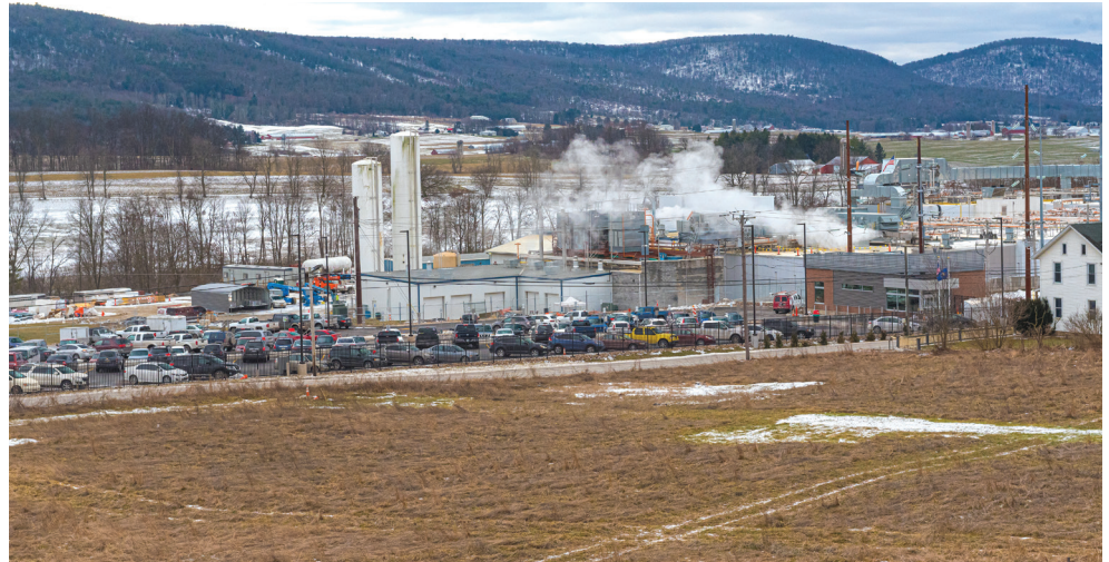
The tract of land just north of the plant awaits construction of the Sustainable Resource Facility (SRF), a comprehensive waste treatment facility that will include anaerobic digesters, an advanced wastewater treatment facility, and a complete organic waste-to-energy facility.
